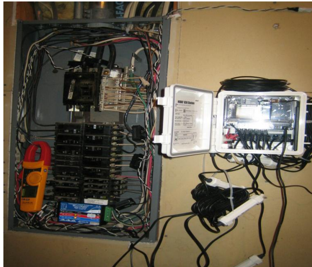
Figure 1: Site Metering Installation
