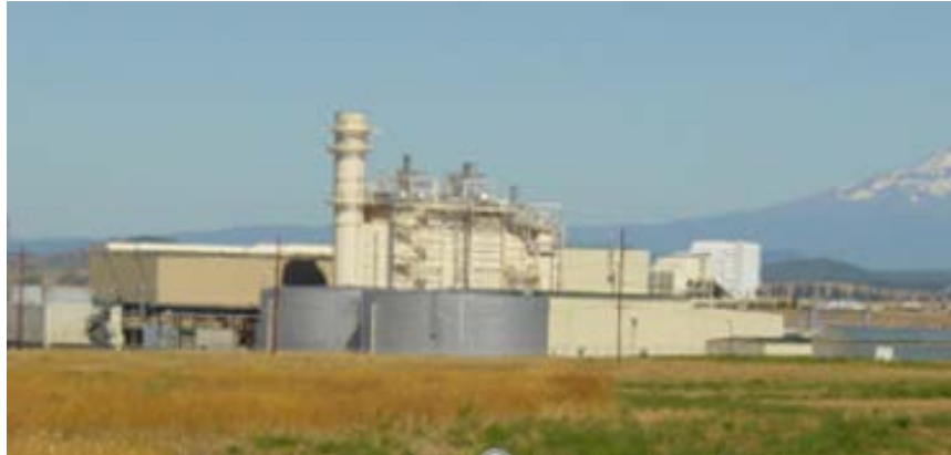
Goldendale Generating Station
