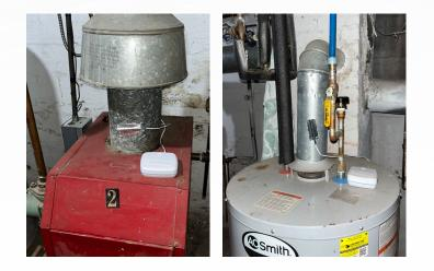
Exhaust duct temperature logging using Lascar surface temperature loggers
