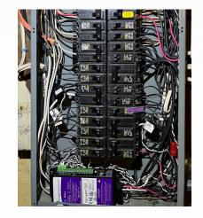
Electric component operation using eGauge in the electric panel (furnace fan, boiler pumps, exhaust/blower fans, dryer use)
